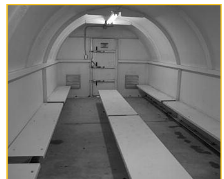
Walker County Commission Storm Shelters
